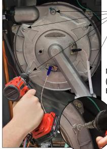
Remove the five M6 nuts from the Burner Door retain these nuts for later reinstallation.
