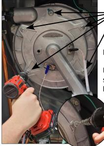
Remove the five M6 nuts from the Burner Door retain these nuts for later reinstallation.
