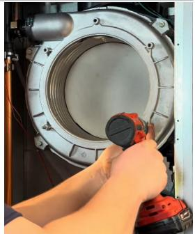
Set the cordless drill/driver (do NOT use an Impact Driver) to the highest torque setting (but NOT to 'DRILL').
