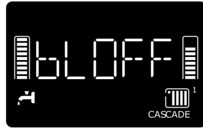
Figure 11 - Master Homescreen 3 - Boiler Off
