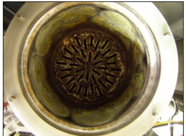
Dirty Combustion Chamber (TFT model shown)
