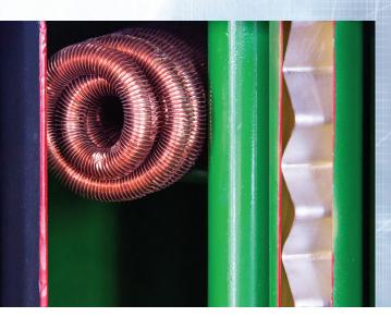
The hot water in the boiler is used to heat cold domestic water as it passes through the coil, heating the water as it is used, or on-demand.
